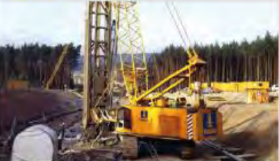
Brombach Main Dam, Germany
