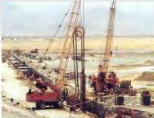
Shwail Dam, United Arab Emirates
