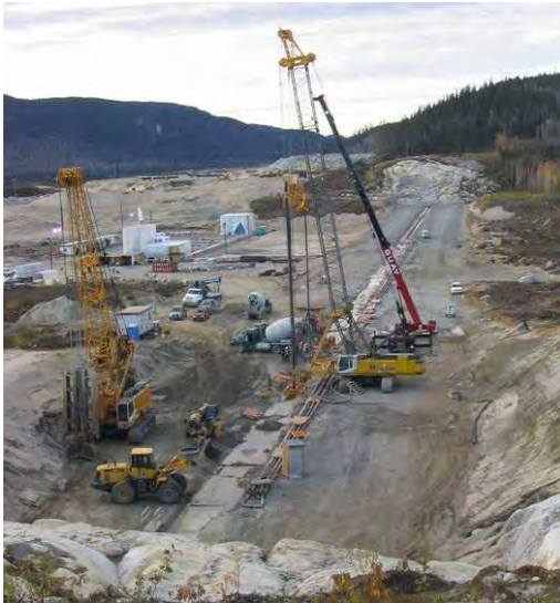
Peribonka Dam, Canada
