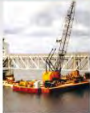
Kingsley Dam, USA
