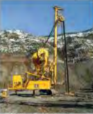
Borcka & Muratti Dams, Turkey
