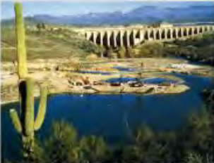
New Waddell Dam, USA
