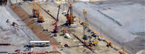
Paribonka Dam, Canada
