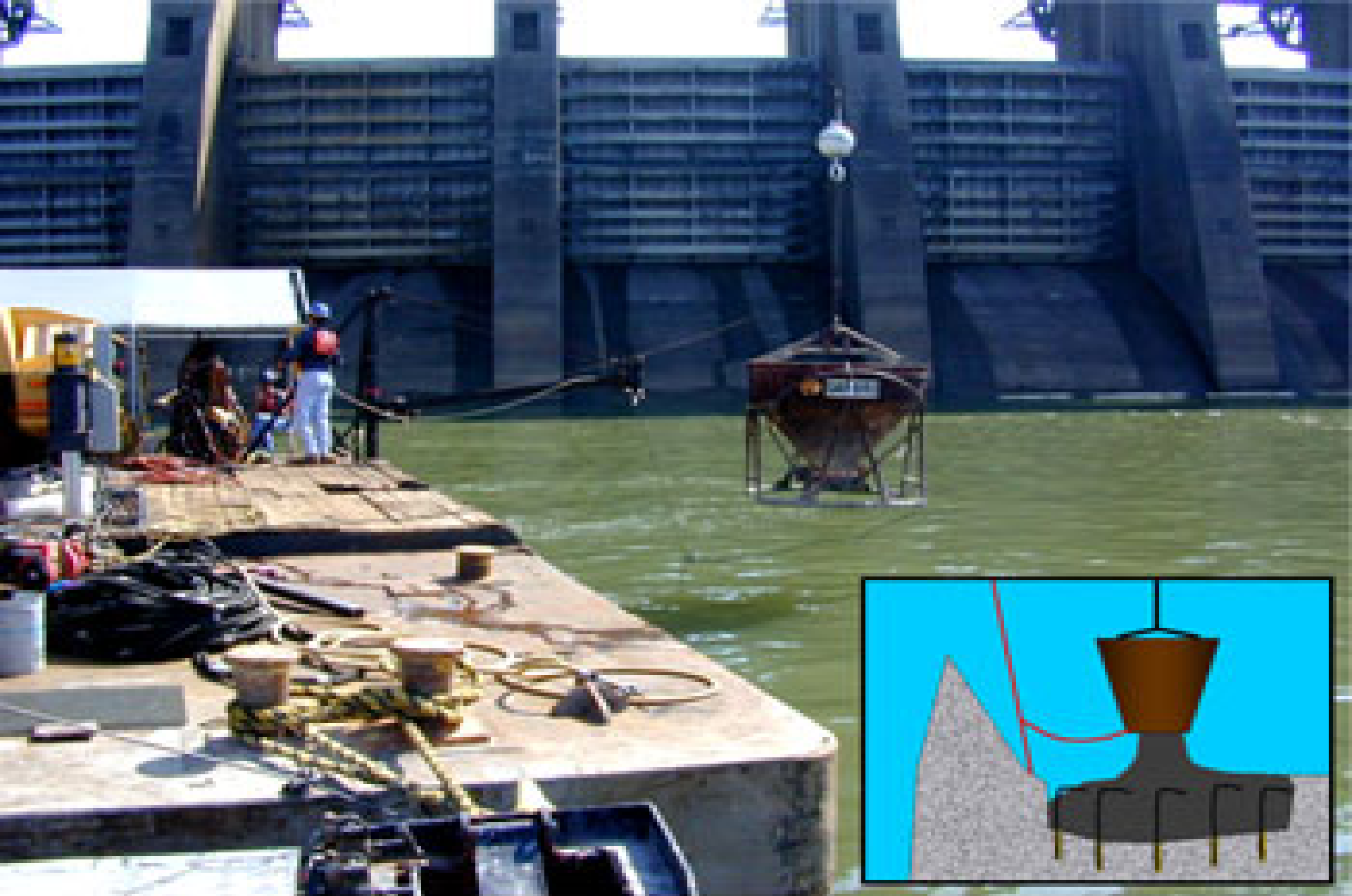
Figure 4 – Placing concrete by bucket. Inset shows guide cable.
